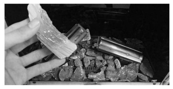
Place log D on the burner tray base at the back of the fire as shown in this picture.
