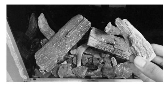
Place log G on the burner tray base at the back of the fire as shown in this picture.
